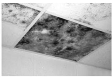
densation at cold surfaces in the occupied spaces such as supply air diffusers or surrounding ceiling tiles. Constant volume systems (such as single-zone or multi-zone systems) are most susceptible to this problem since they modulate supply air temperature in response to changes
