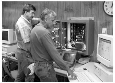
Shawn Bodkins (left) and Darrell Cimbanin in Fort Hood's DPW work on multiple workstations for HVAC controls that will all be tied to a single workstation.
